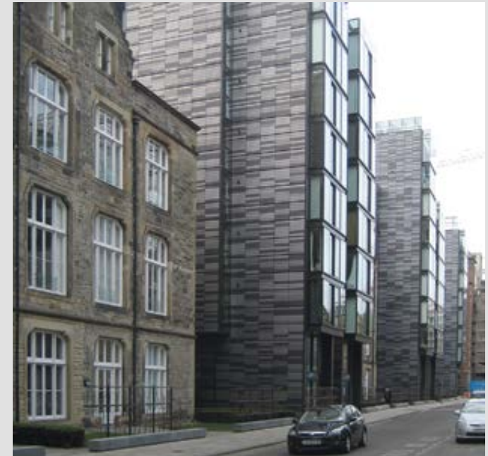
Aluminium—Simpson Loan Multi-toned anodised aluminium cladding provides a striking and positive contrast to the historic buildings making the distinction between new and old very clear.
