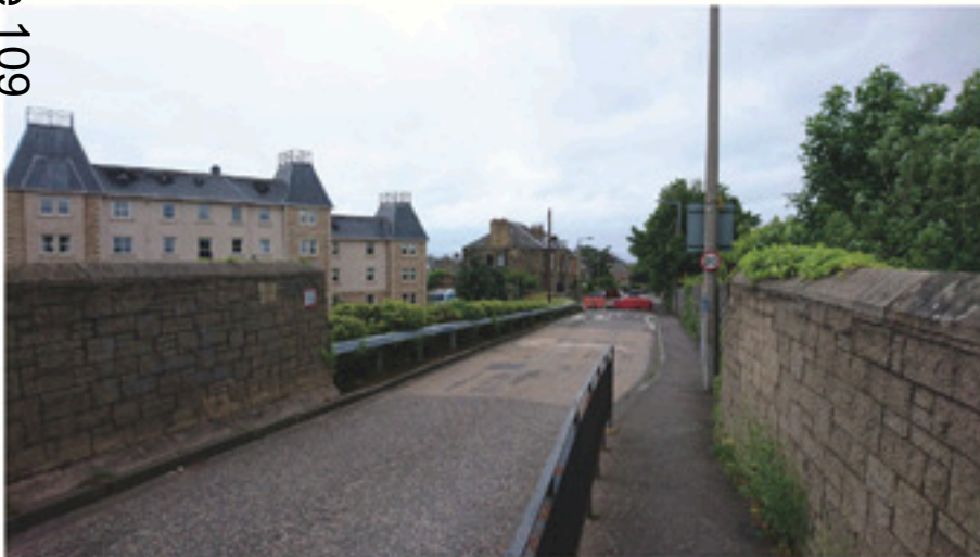
View North, looking down Brunstane road, over railway bridge. New build flats to the left. More two storey town houses continue towards Portobello High St.
