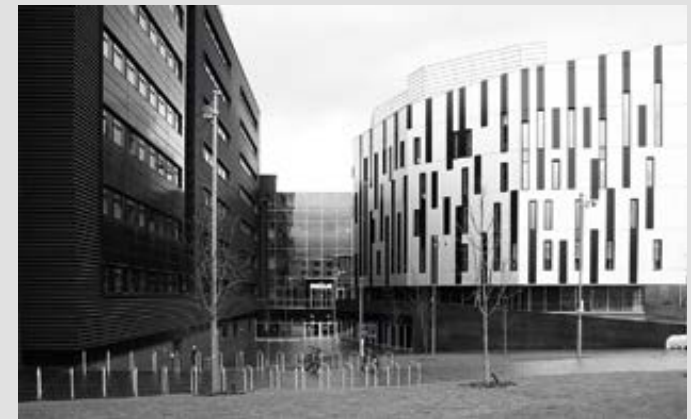
High quality detailing—Sighthill Court Construction of a sample panel and approval were required by condition in order to ensure the design intent of a high quality finish was executed.
