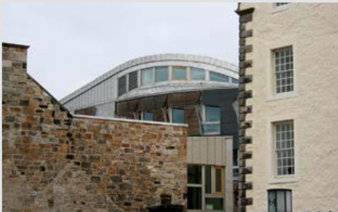
Metal roofing in a historic context—Canongate Stainless Steel roofing has been used on the Scottish Parliament.
