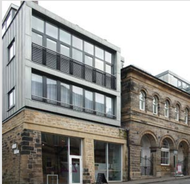
Using zinc to provide striking contrast—Infirmiry St. The zinc cladding combined with the modern building form provides a positive contemporary contrast to the historic former Infirmiry Street Baths building.
