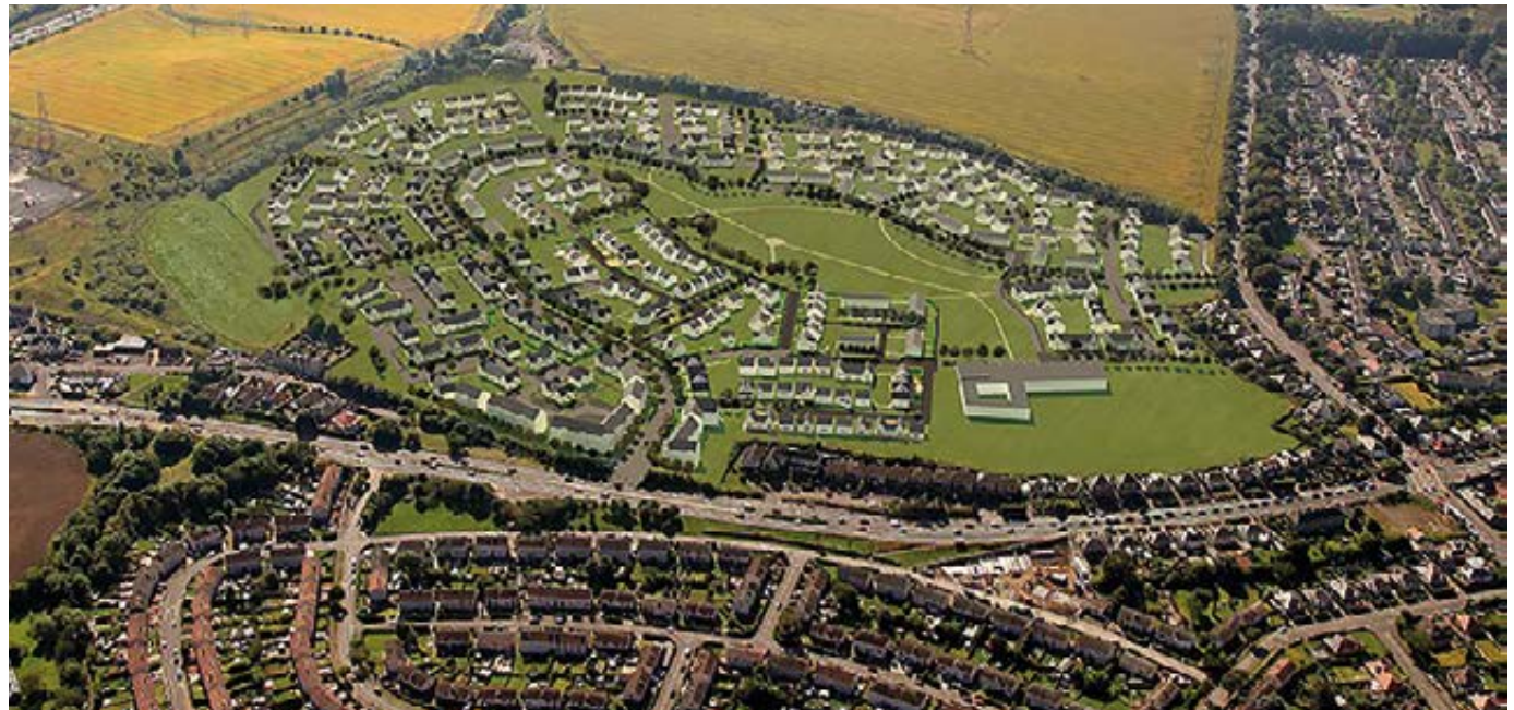
Aerial view of Broomhills Park (Barratt East of Scotland Ltd)
