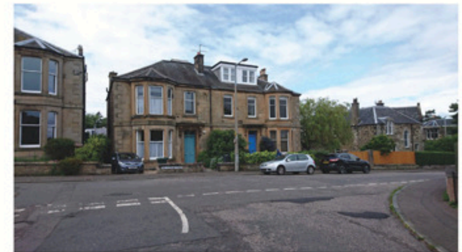
16 Brunstane Road, two storey town house with front facing dormer, wider than non-statutory guidelines allow.
