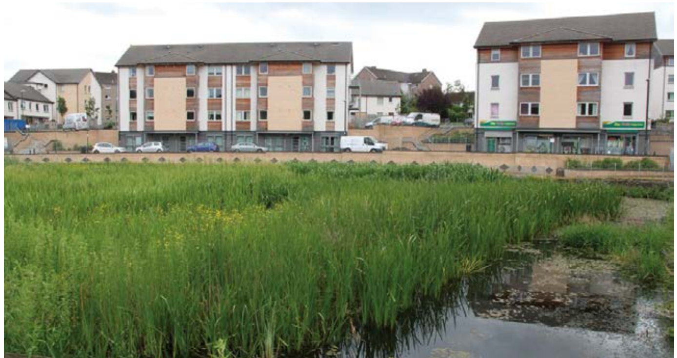
SUDS retention basin, Firrhill Neuk, Oxgangs
