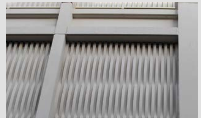
Textures created with concrete—Princes Street Concrete panels with a textured surface treatment are used on this recent building on Princes Street.
